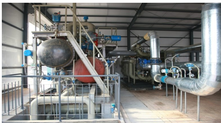
Figure 2: Test for electricity generation based on middle-low temperature geothermal energy in Huabei oilfield.
