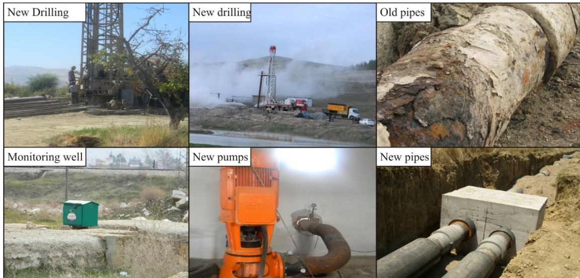
Figure 5: New production, reinjection and monitoring wells and new pumps-pipelines from Omer-Gecek field.
