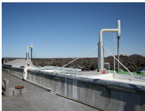
Figure 2. Silica sedimentation tanks at the Blue Lagoon
