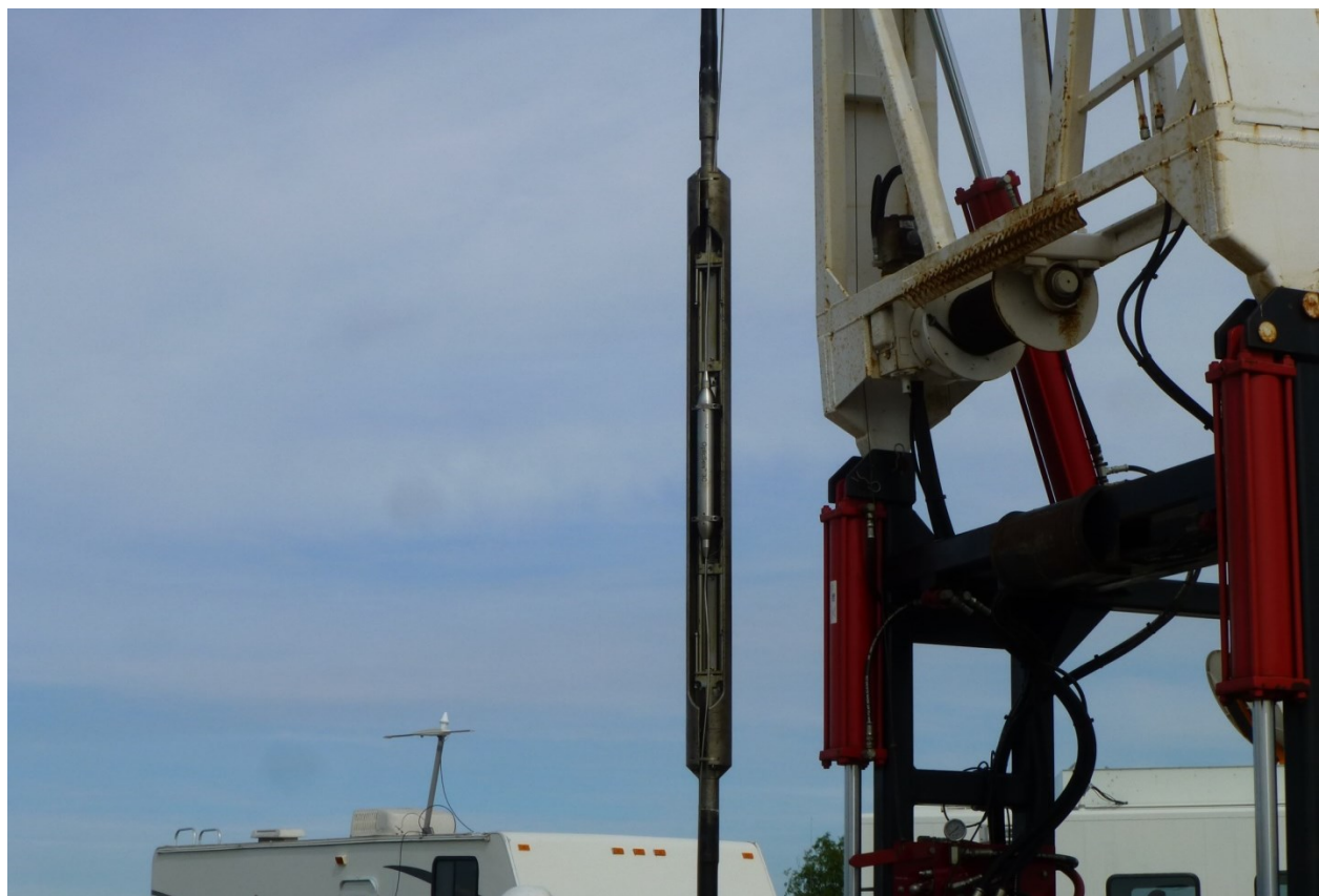
Figure 16. One of the sensor pod housings with the fiber optic sensor pod attached prior to lowering the assembly into the well.
