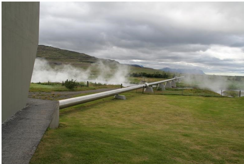
Figure 10: Pump station at Deildartunguhver and a pipeline feeding the hot water to villages Borgarnes and Akranes some 70 km away from the spring. This is probably the longest hot water pipeline for space heating in the world.
