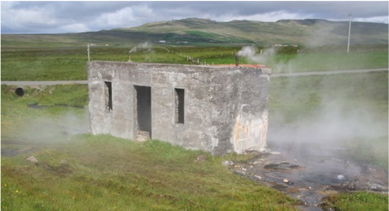
Figure 7: House made of concrete by Hurdarbak in Borgarfjörður W-Iceland, built around 1900. In the right part is a kitchen with stove made of concrete. Steam from the boiling spring just right of the house was piped into the house and heated the stove. In the left part are facilities for washing clothes.
