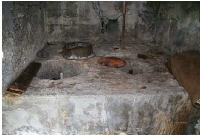
Figure 8: The concrete stove in the Hurdarbak kitchen house. There are holes for three pots.
