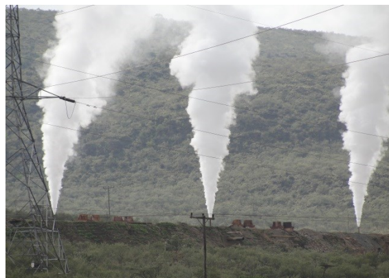
Figure 2: OW 44 series discharging. The wells have a discharge a combined capacity of 20MW
