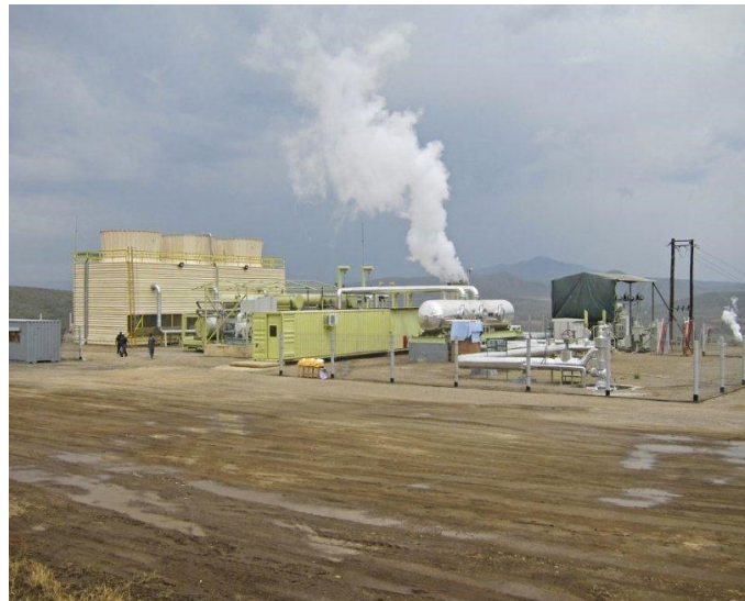
Figure 5: the 2.5MW Olkaria wellhead generator
