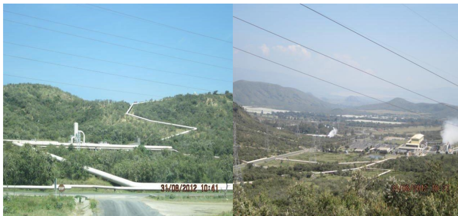
Figure 6: photos showing the long steam lines delivering Steam to the conventional Olkaria II power plant
