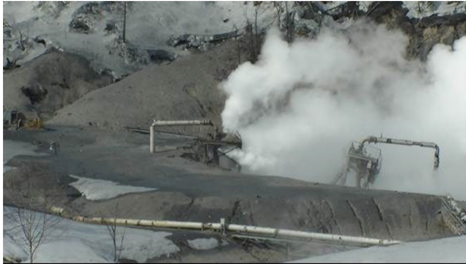
Figure 7: Steam leaking through casing head just under the closed well head valve of the Well 138 (on 9 March 2012)
