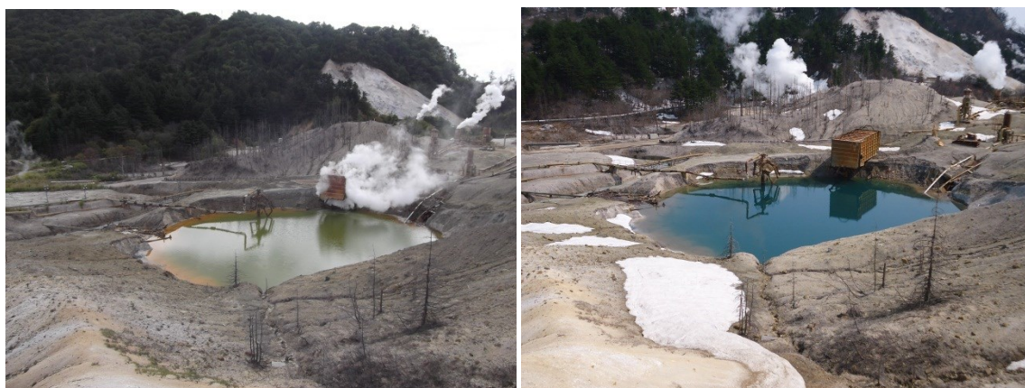
Figure 10: Change of steam leakage from Well 138 before relief well affected (left; 26 September 2013) and after (right; 18 April 2014)
