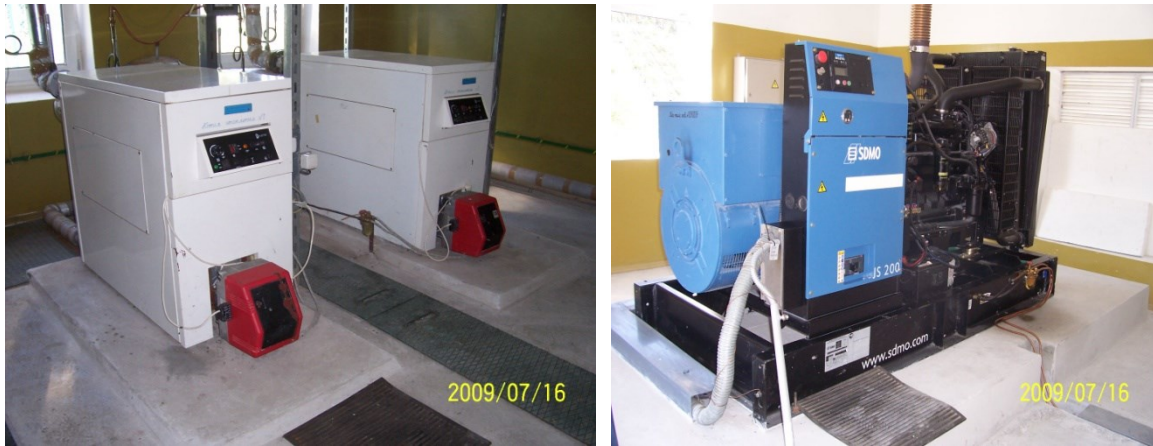
Figure 6: Two reserve liquid-fuel boilers and a diesel electric generator at the Frontier point “Novaya Rudnya” in the Elsk District, Gomel Region.
