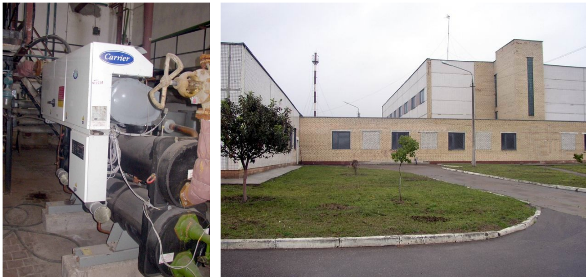
Figure 7: Heat pump Carrier 30HXC110 (to the left) in the process of its installation at the sewage header building No.24 in Novy Dvor, Minsk District (to the right) [Zui, Martynova, 2013].
