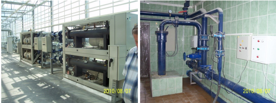
Figure 2: Two heat pumps Daikin EWWD 440MBYN at the Greenhouse Complex “Berestye” in the vicinity of Brest town (left) and the wellhead assembly of the Vychulkovskaya 201 borehole.
