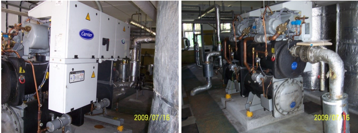
Figure 4: Heat pump of the model Carrier Global Chiller 30HXC 080-375 at the Frontier point “Novaya Rudnya” between Belarus and Ukraine in the Elsk District, Gomel Region [Zui, Pavlovskaya, 2012].
