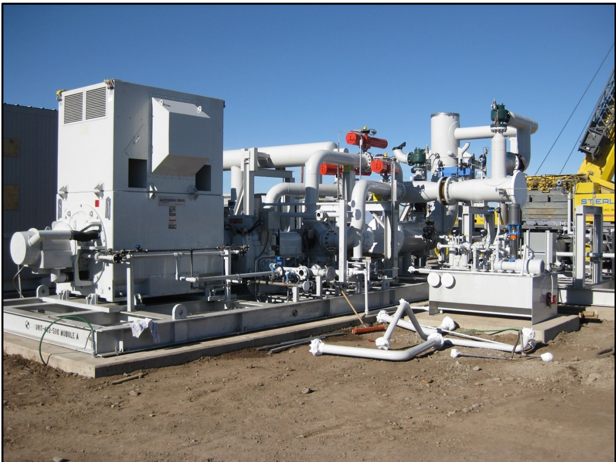
FIGURE 8. Photograph of the Paisley Power Plant generator, turbine, heat exchanger, and condenser piping.
