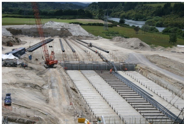
Figure 8 - Pulling 100 m lengths of pipe into position
