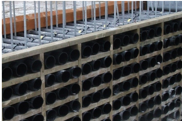
Figure 9 - Head chamber construction before casting into wall
