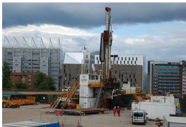
Figure 1: Drilling of the Science Central Borehole in the centre of Newcastle-upon-Tyne. (Credit: British Geological Survey)
