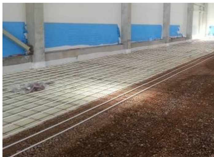
Figure 17: The view of floor heating system installation in the logistic center.
