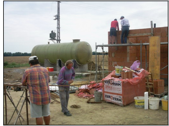
Fig. 8. – Construction of pump house and the 20m 3 water tank made of fibreglass polyester
