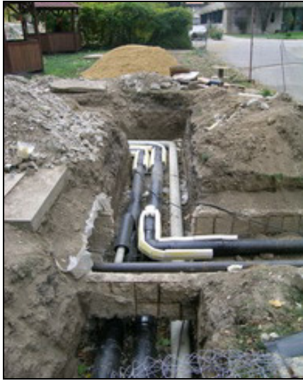
Fig. 7. – Part of the three pipe system
