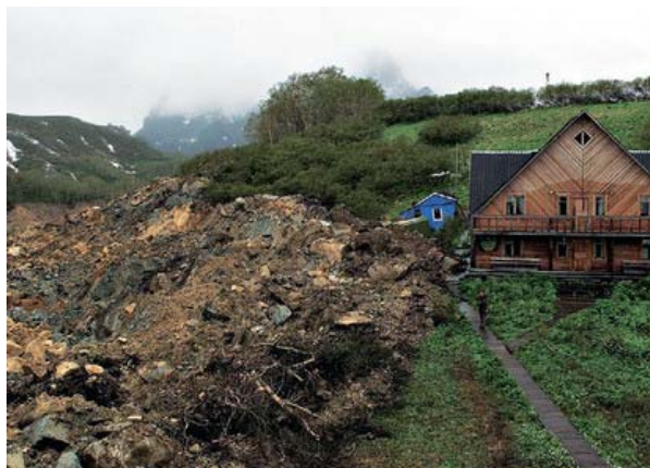
Figure 3: Large-block avalanche body near buildings of Kronotskiy Biosphere Reserve in the Valley of the Geysers. This is an example of the negative effects of natural disasters on constructions built without taking certain dangerous phenomena into consideration. Photo by S. Gorshkov (National Geographic). June 22, 2007.
