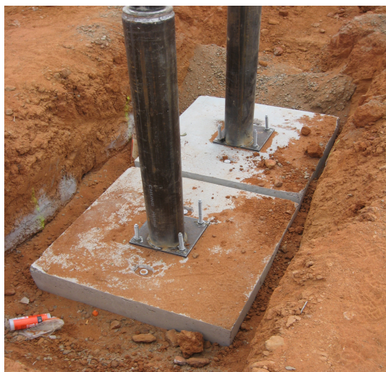
Figure 4: Typical pipe support footing.
