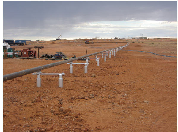
Figure 3: Pipeline under construction.
