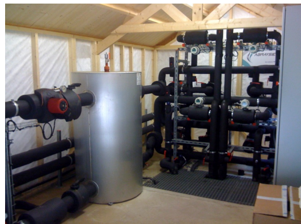
Figure 3: Equipment of one horizontal ground heat exchanger sector with 2 fluid loops at 1 m depth
