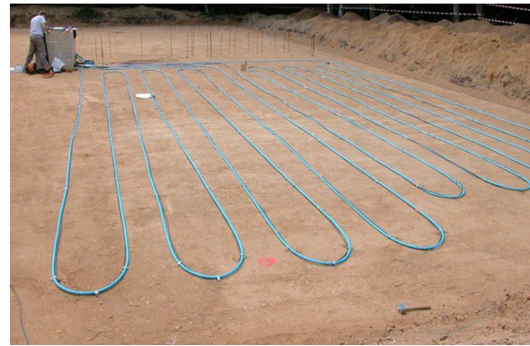
Figure 3: Equipment of one horizontal ground heat exchanger sector with 2 fluid loops at 1 m depth
