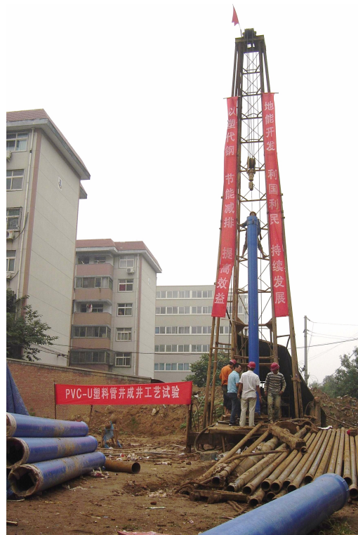
Figure 4: Photograph of PVC-U Tube Sinking Process
