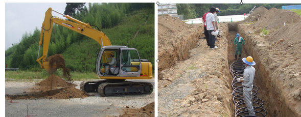
Figure 4: Excavation of trench (left) and laying of slinky coils (right).
