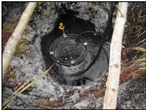
Figure 8: Downhole Heat Exchanger in Natural Geothermal Well
