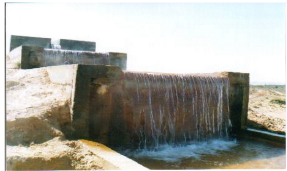
Figure 3: The water cooling system (Cascade of Oum Elfareth locality, Kebili area)
