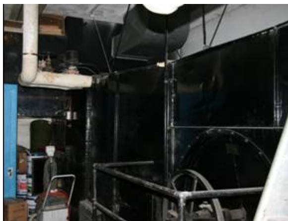
Figure 6. One of the two large force air units supplying heat air to the auditorium and supplemental heat to the classrooms.
