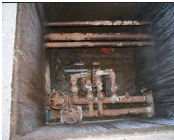
Figure 5. Roosevelt geothermal well with two 6.4-cm diameter downhole heat exchangers. The pipes in the upper part of the photo are connected to the second well.
