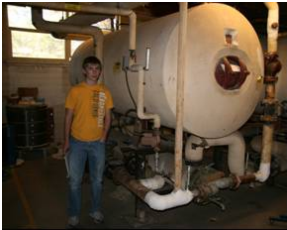
Figure 8. One of the three former oil fired boilers used as a storage tank for the heated secondary water at Ponderosa Middle High School.
