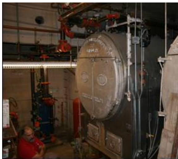
Figure 13. Main plate heat exchanger and hot water boilers for Klamath Union High School.
