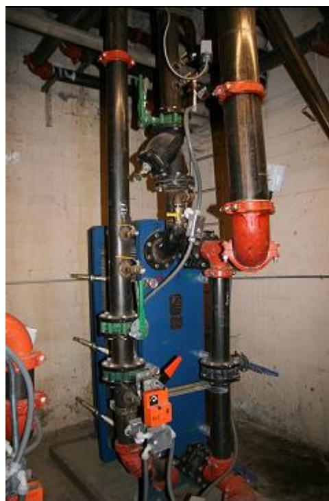
Figure 14. Detail of the main plate heat exchanger at Klamath Union High School.
