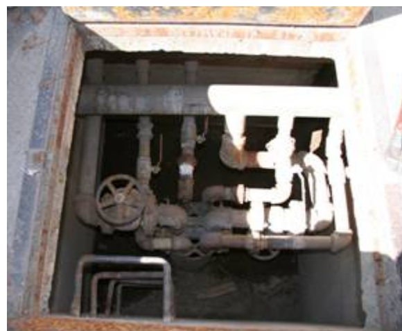
Figure 7. Downhole heat exchangers at Ponderosa Middle School: 2@5-cm and 1@ 7.5-cm diameter feeding into a common header.
