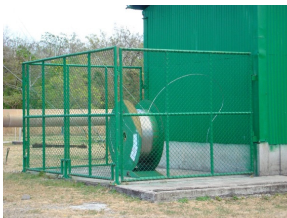
Figure 12: Spool with capillary tubing. Photo by P. Moya.
