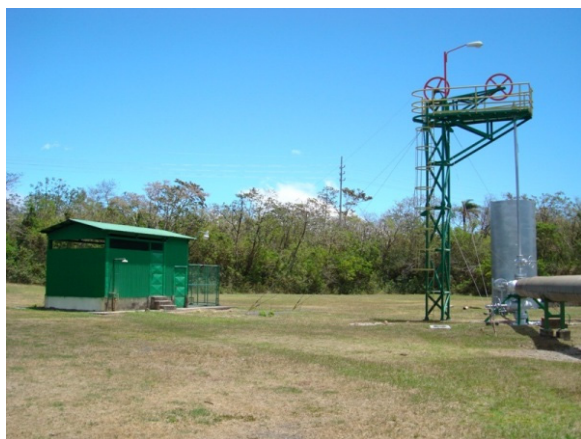
Figure 5: The calcium carbonate inhibition system at well PGM-03. Photo by P. Moya.
