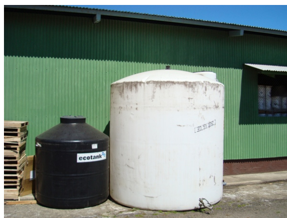
Figure 6: Inhibitor storage tanks. Photo by P. Moya.
