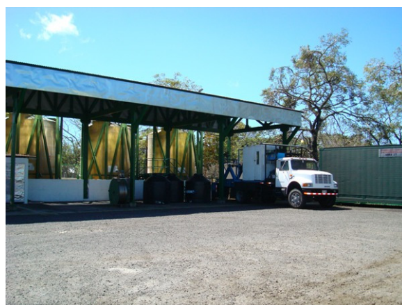
Figure 6: Inhibitor storage tanks. Photo by P. Moya.
