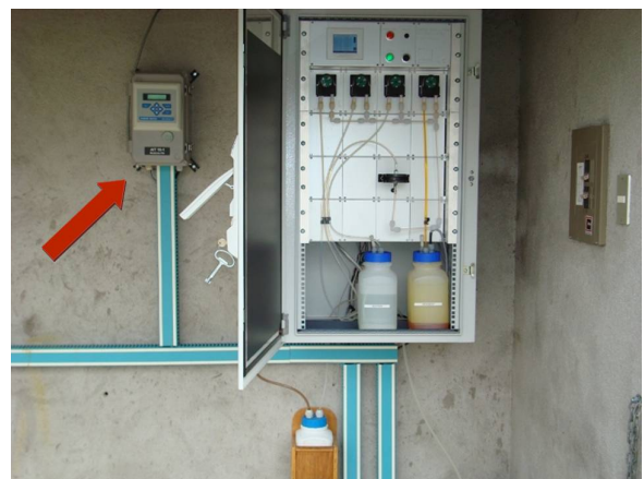
Figure 14: pH instrument for continuously record pH values. Photo by P. Moya.
