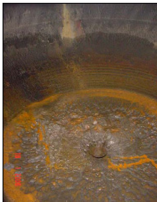
Figure 9: Deposit on scrubber bottom.
