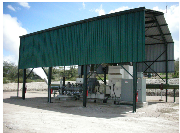
Figure 2: Steam Turbine and Gearbox Being Installed at Oserian’s Facility
