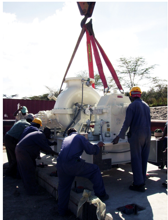
Figure 2: Steam Turbine and Gearbox Being Installed at Oserian’s Facility
