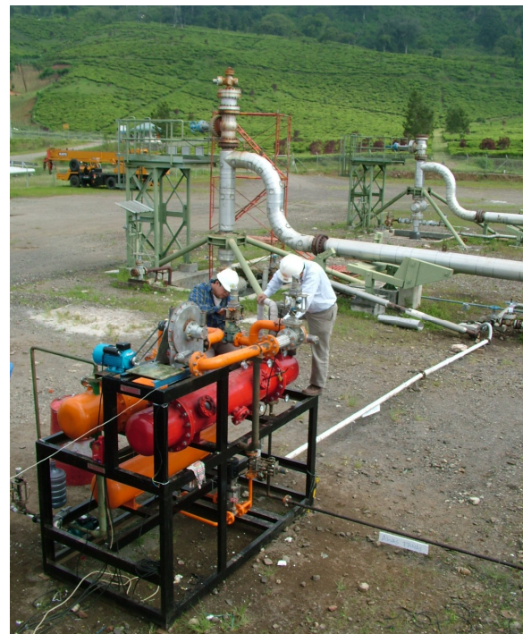
Figure 15. Assembly of 2 kW binary cycle plant at Wayang Windu
