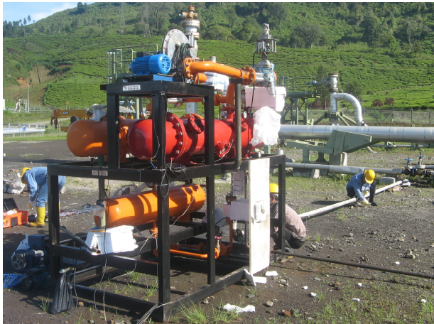
Figure 15: Installation of the binary cycle geothermal power plant model
