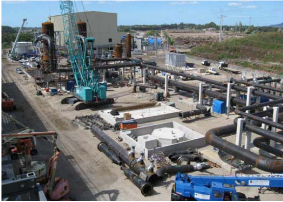
Figure 2: Feb 08 - View from the south-east edge of the cooling tower showing the extent of the mechanical erection in the steam separation area.
