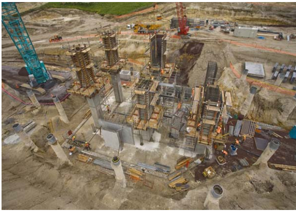
Figure 1: Aug 07 - Aerial view of the Powerhouse Structure depicting the 'vertical' range of activities from the 14m deep U-Seal pit to the 25m high roof structure.
