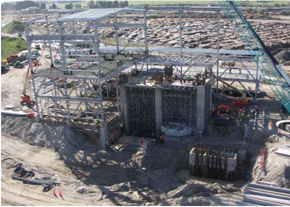
Figure 1: Aug 07 - Aerial view of the Powerhouse Structure depicting the 'vertical' range of activities from the 14m deep U-Seal pit to the 25m high roof structure.
