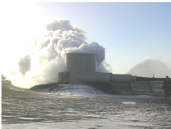
Figure 6: Wellhead vertical drum silencer (from Dr. Bjarni Pálsson, 2007) ( staff.unak.is/not/hreidar/MAU1103/Djupboranir.ppt )
