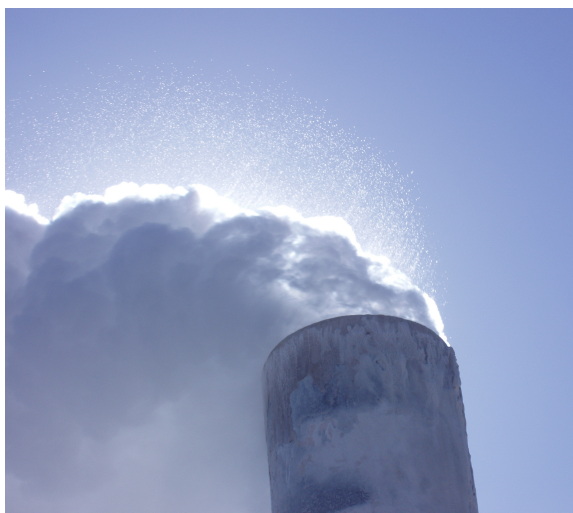
Figure 5: Here we see a very unfortunate result of a silencer design. Big, salty, silica laden drops are thrown out of the silencer steam exhaust stack.
