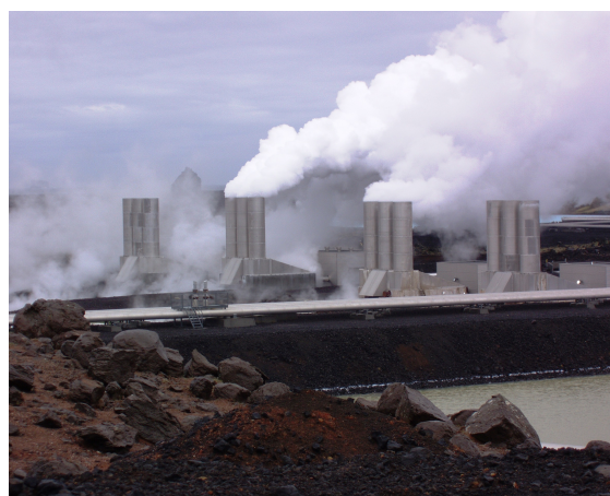
Figure 1: The Reykjanes separators silencers
