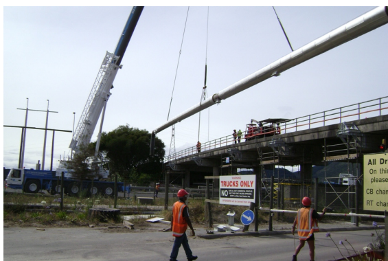
Figure 13: Lifting the 55m pipe onto the bridge over the State Highway
