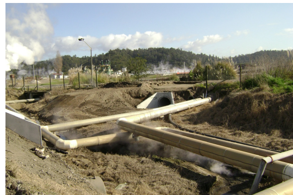
Figure 14: Running new pipes over old in a tight spot
