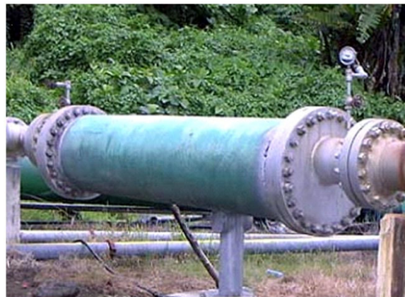
Figure 3: The original 1R8D solid trap installed.
