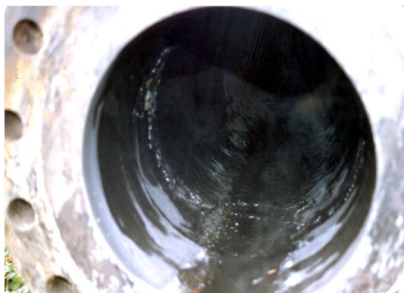
Figure 6: Minimal debris collected at the main brine line even after the installation of the new modified solid trap.
