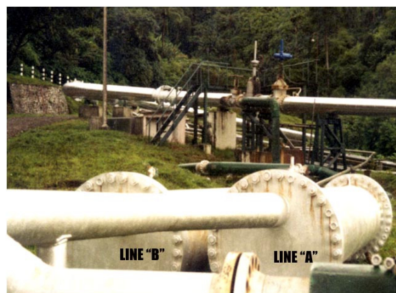
Figure 4: The new 1R8D modified solid trap installed.
