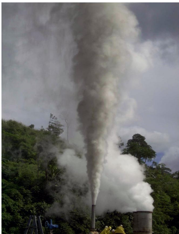
Figure 2: Well 1R3D clearing discharge showing some dark debris being ejected.
