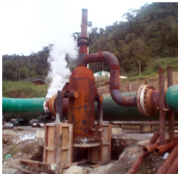
Figure 5. The two-phase strainer installed in a production well suspected of contributing solids. The strainer reduced the power output of the well by 1-2 MW and was subsequently removed.
