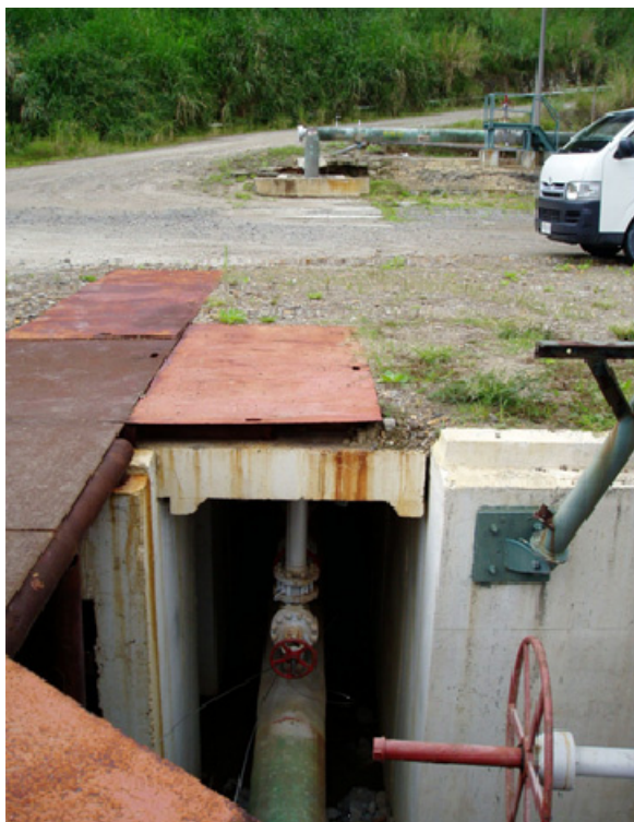
Figure 6. The original location of Pad C MBL solids trap in a deep cellar. The trap was only 18" in diameter and produced a fluid flow that was not effective in capturing large amounts of solids.
