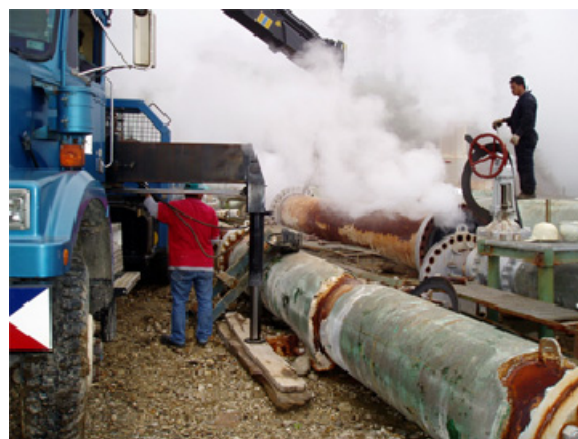
Figure 8. Maintenance crews conduct regular monthly cleaning and inspection of the traps to maintain its efficiency.
