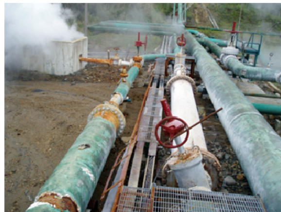
Figure 7. Above shows the location at pad surface of the two 30"-diameter solids trap modification from the original set-up. Adding a redundant solids trap allows cleaning of one solids trap at a time without affecting continuous brine injection.
