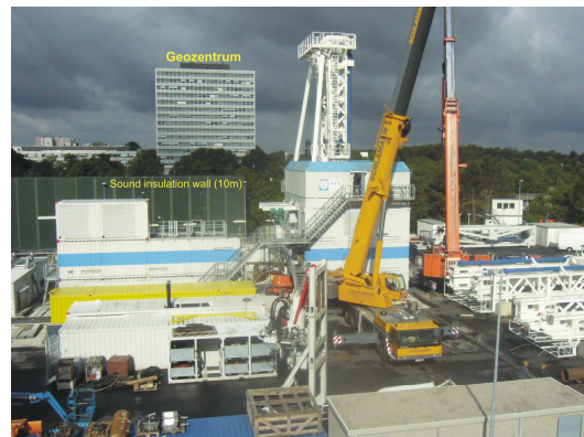
Figure 6: Photograph of the drill site in Hannover on June 12, 2009 during rigging up the InnovaRig
