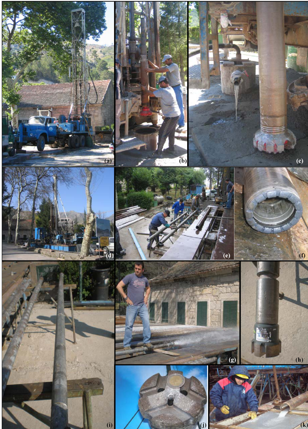
Figure 7: Images of the perforation techniques used in the construction of US1 probing, by rotopercussion system (a, b, c), by system of rotation with continuous rotation of the drill core (e, f, g) and with guided perforation system (g, h, i, j, k), in Unhais da Serra, Portugal. Note: the system of guided perforation adapts to the continuous rotation of the drill core, with the detail of substituting the classic head and gauge for a hollow bar (i) in association to a piece with a gentle curve before the bit (h); bit rotation is triggered by an iron rod of helical shape in the interior of the hollow bar so that receiving injected water at high pressure (g) causes the rotation of the bit; thus, because the only things moving are the interior of the equipment and bit, it is possible to control the deviation curve position in the interior of the hole. Also note the fact that in the classic continuous rotation of the drill core, the head spins in harmony with the rods and with the head of rotation on the surface.
