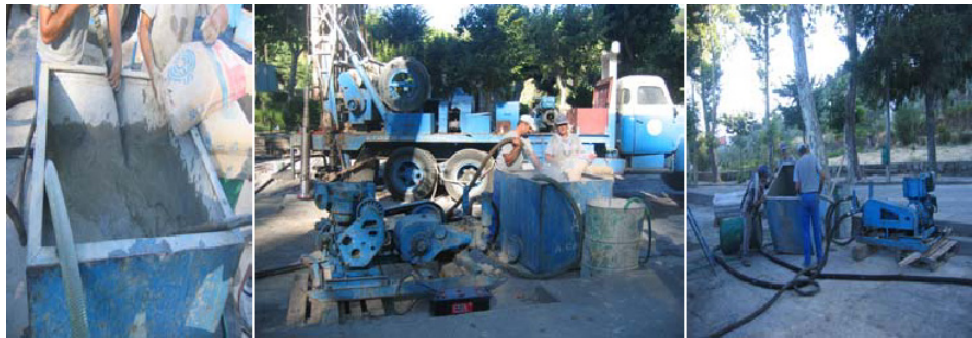
Figure 9: Images of manual preparation of syrup (cement grout) in recipient and of pump for injection in the interior of the drill US1, in Unhais da Serra
