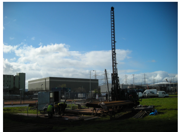
Figure 10: Drilling the GSNI Kilroot borehole. Picture T. Rosowski
