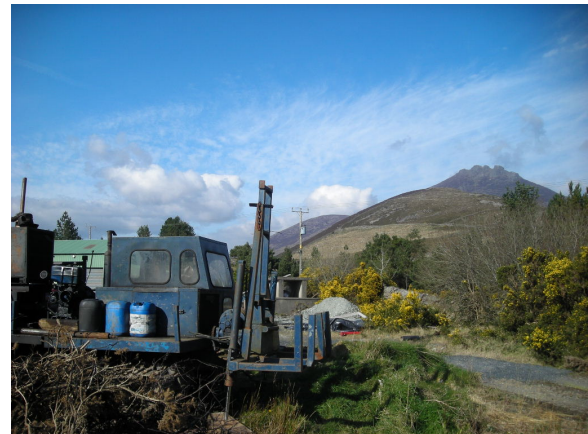
Figure 14: Setting up the GSNI drill rig for the Mourne granite assessment borehole. Pic T. Rosowski
