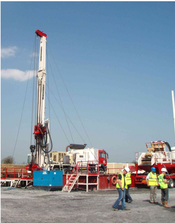
Figure 12: GT Energy's Marriott rig exploring a fracture aquifer south-west of Dublin.
