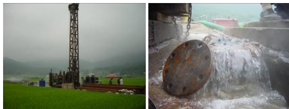
Figure 6: Drilling rig (left) and overflowing geothermal water from BH-2 (right)
