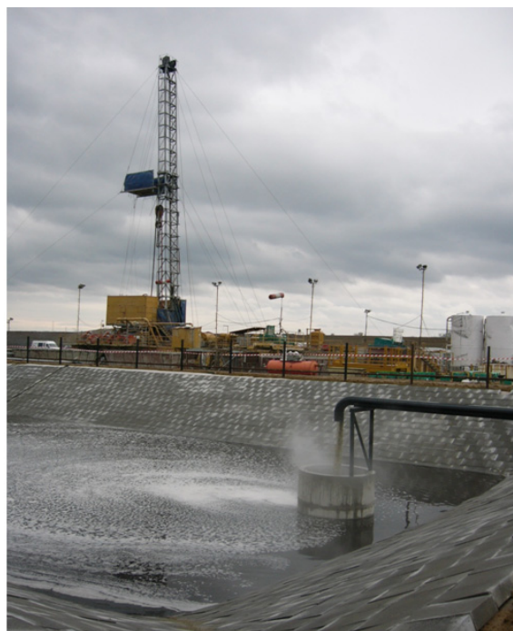
Figure 2: Testing existing hydrocarbon wells in southwestern Hungary
