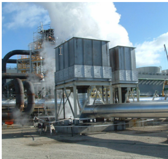
Figure 6: High Pressure and Low Pressure Silencers in Operation during plant startup.
