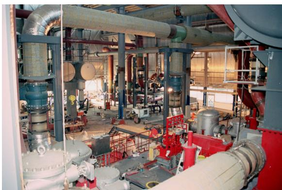
**PP-6:** PP-6 inaugurated in December 2007 comprises one single flow, triple steam inlet (16/6.5/1.2 bar) 30 MW<sub>e</sub> turbine generator manufactured by Fuji Electric Systems.
