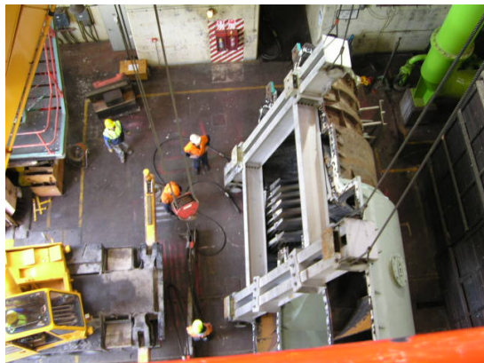
Figure 10 - Photograph of Top MP casing rolling frame in use in 2008
