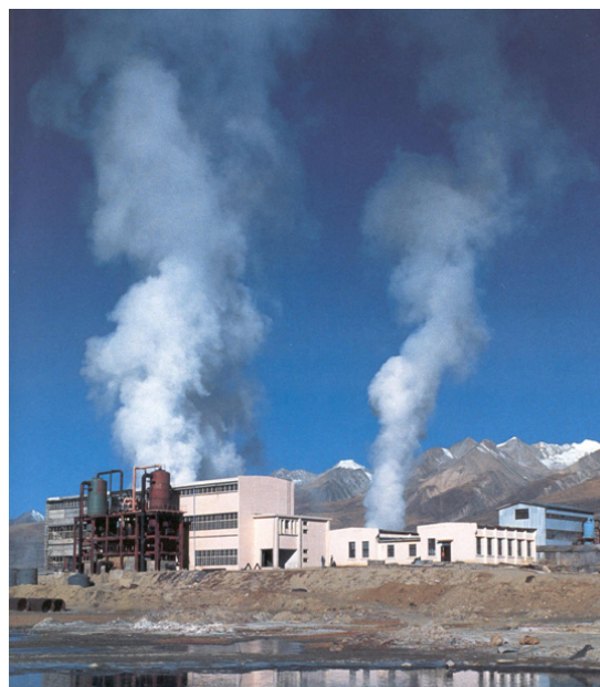
Figure 1: Geothermal power generation in Yangbajain
