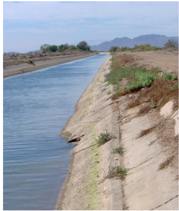
Figure 4. The Cerro Prieto fault crossing an irrigation channel at F3 (Fig.1).
