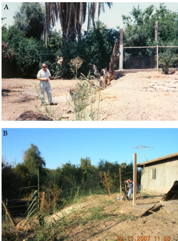
Figure 2. Photograph of site F1 (Fig.1) showing the Saltillo fault where the crackmeter is installed as seen from the South. This place was flat in the beginning of the 1970s. A) Photograph taken in 1994. B) Photograph taken in 2007.
