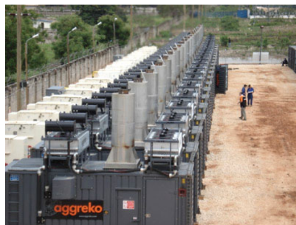
Figure 5: Containerized gensets from Aggreko for Emergency power (temporary measure).
