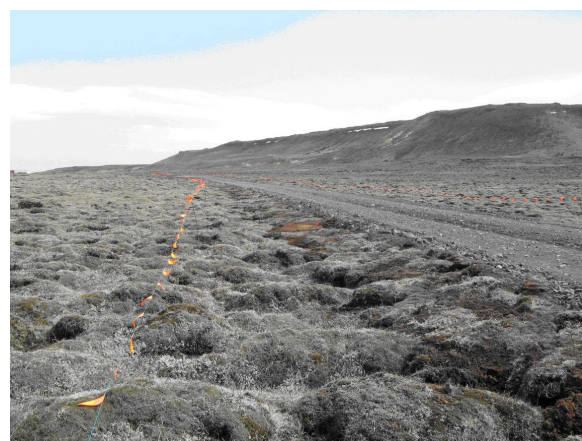
Figure 10: Access road to a drilling platform. The vegetation which had to be removed from the ground is led at the side of the road during construction. The flagged line on both side of the road determines the construction area.
