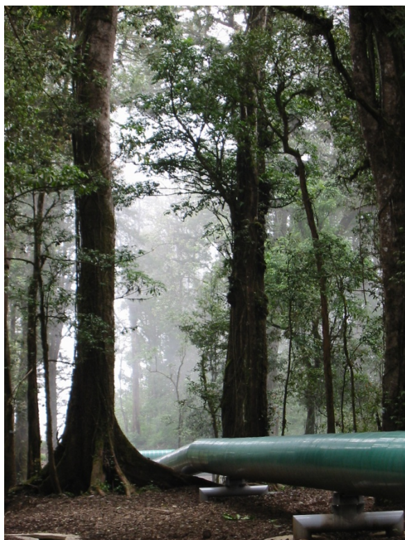
Figure 1: A green pipeline at the Darajat geothermal project. Note the buttress tree root extending under the pipeline
