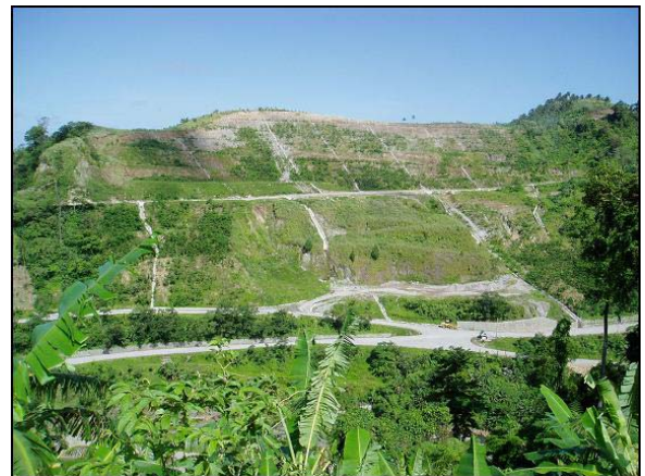
Figure 17. Photo showing slope modification implemented at the 105 Mahiao slide area.
