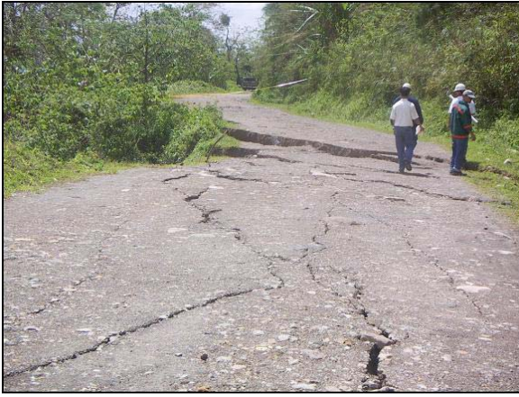
Figure 9. Photo shows cracks along the upper road within the slide area.
