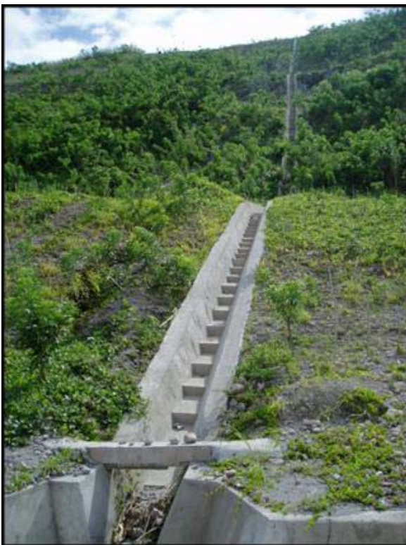
Figure 16. Photo showing concrete-lined ditches designed to address surface run-off in the slide area.
