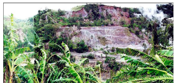
Figure 5. Photo taken last 2001 showing minor benching undertaken to address the landslides after Typhoon Auring.
