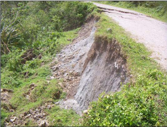
Figure 10. Smaller slide scars noted beside those cracks along the upper road.
