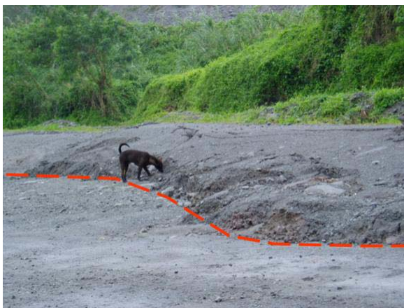
Figure 7. Pressure heaves or bulges found at the lower road which appeared at the same time when cracks were observed at the upper road after a period of continuous rains in the project site.
