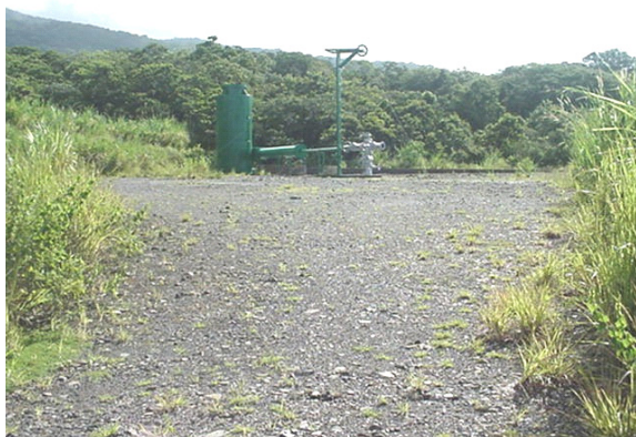
Figure 18: Work site after recovery activities (Pailas).
