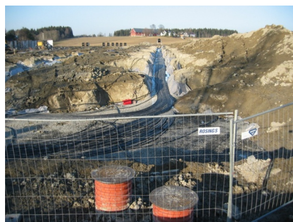
Figure 3: The BTES at Ahus under construction in summer 2007 (Photo: Forum Fjernvarme).
