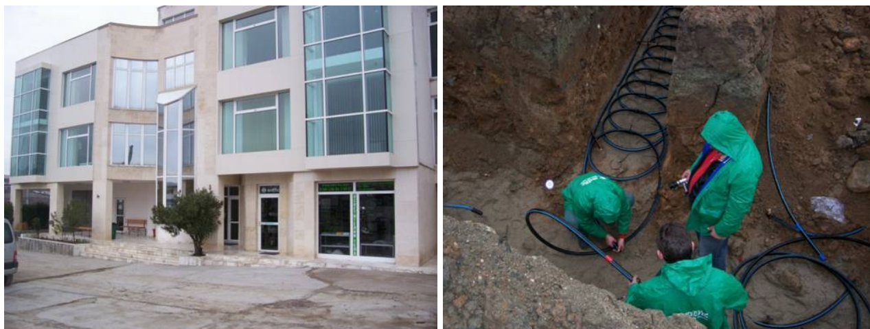
Figure 8: GHP heating and cooling of an office building (Sandanski town, SW Bulgaria) (heating capacity - 22,5 kW, cooling capacity- 25,0 kW)
