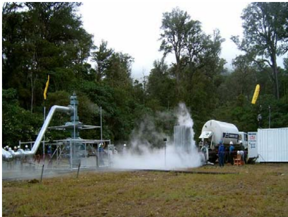
Figure 7: Pumping Nitrogen into the well BEL-03.
